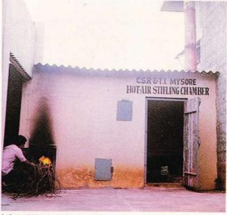
The front view of 'Ushna Kothi' shows firewood type oven, front door, bottom ventilator, temperature recording place and chimney.
