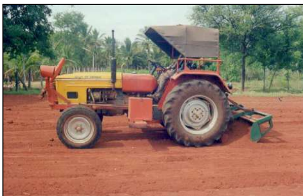
Figure 3.1: Levelling and grading of the field for a new mulberry plantation with tractor operated leveller
