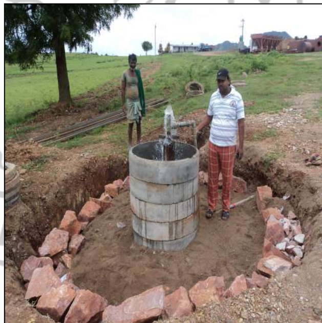
Figure 3.25: Rainwater recharge pit around the bore well
