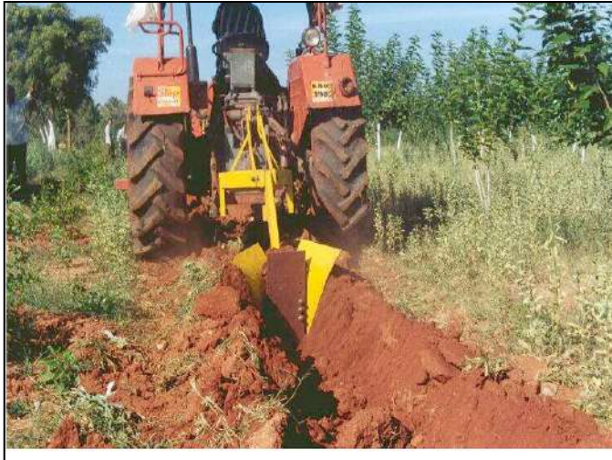
Figure 3.9: Opening of trenches by the trencher
