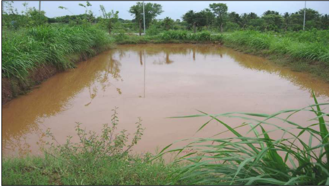
Figure 3.22: Deep pit for runoff collection and percolation
