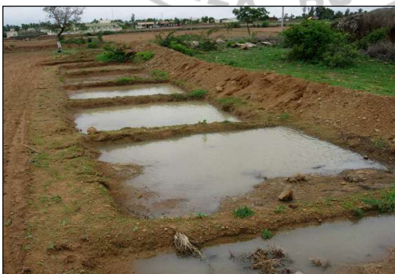
Figure 3.21: Runoff collection pits
