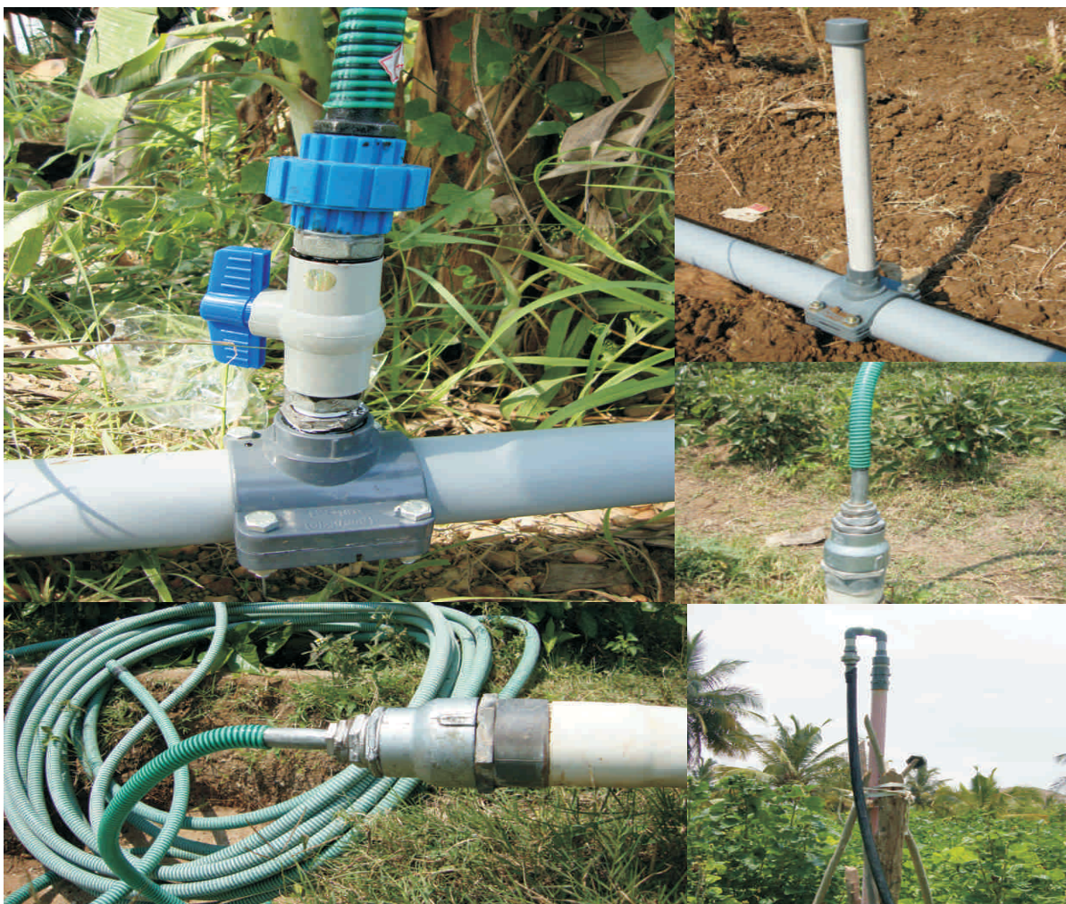
Arrangements for diversion of irrigation water for jetting in mulberry garden to manage papaya mealybug and other sucking pests
